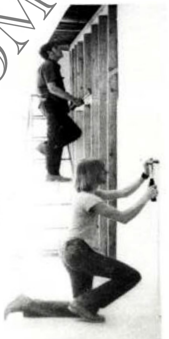
Seniors John Rawlins (on ladder) and Mike Minsker assembling new partition in the cafeteria annex. (Photo by Don Gibson)
